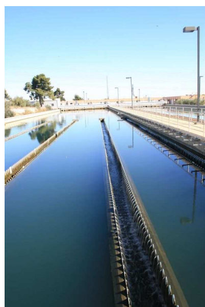
Zai water treatment plant, Jordan, December 2006. Caring for freshwater supply and working against drought.
